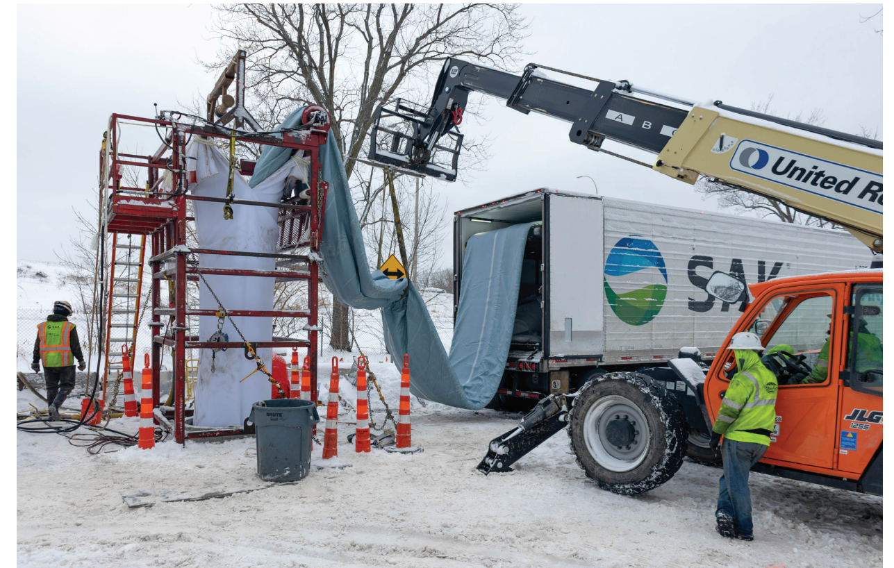
CIPP Lining, Minneapolis
