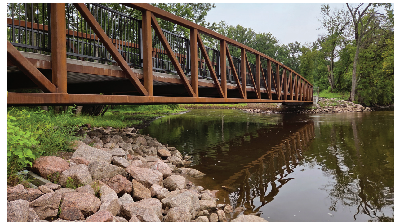
Coon Rapids Stormwater Flood Alleviation
