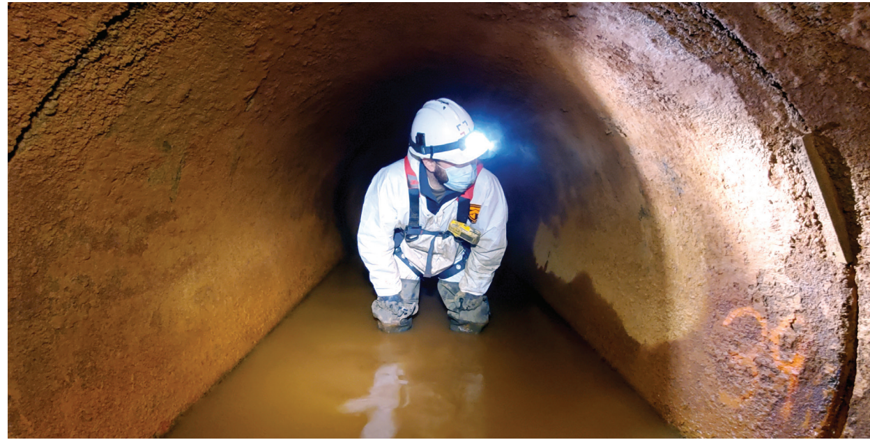
Lake Street Siphon Inspection
