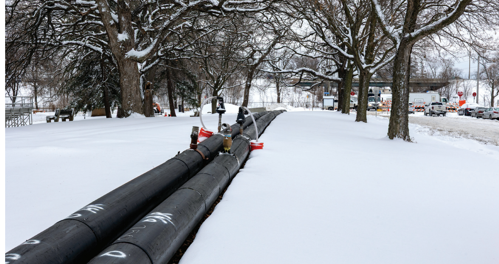
Trenchless Pipe Rehabilitation, Minneapolis
